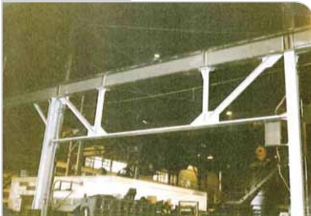
Truss-type reinforcement (example 2).
